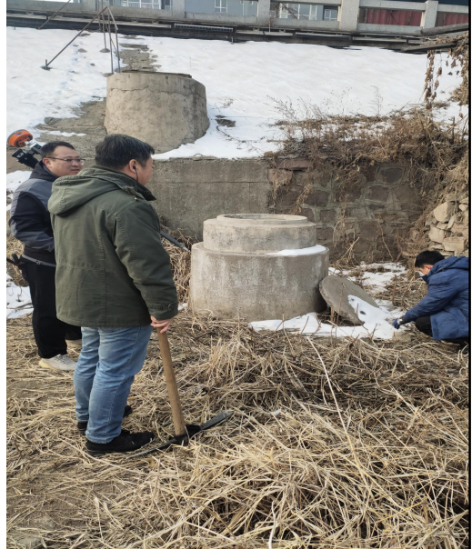
终点处现状污水检查井
